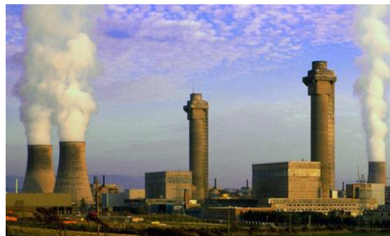
FIGURE 64 Windscale Reprocessing Towers
