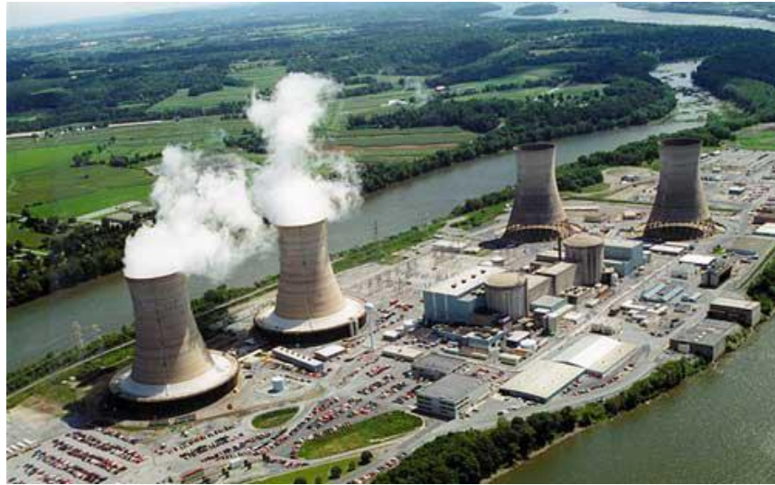
FIGURE 49 Three Mile Island Nuclear Power Plant, U.S.
