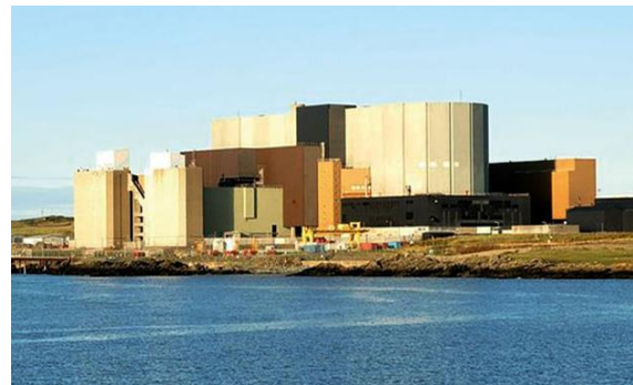
FIGURE 39 Wylfa MAGNOX Nuclear Plant, UK
