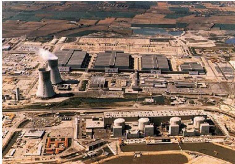
FIGURE 16 French Gaseous Diffusion Plants Located Behind the Two Nuclear Reactor Cooling Towers. Nuclear Reactors Are Needed to Power the Diffusion Plant.
