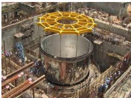
FIGURE 46 India's Prototype Fast Breeder Reactor Under Construction at Kalpakkam
