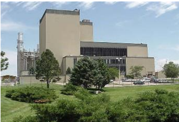
FIGURE 55 Fort St. Vrain HTGR Power Station. It Operated from 1976 to 1989.
