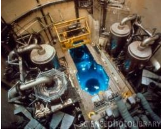
FIGURE 31 Interior of a Nuclear Containment Building During Refueling
