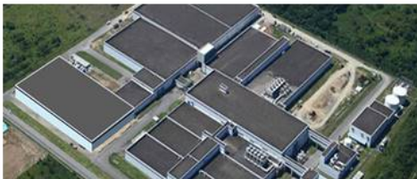
Rokkasho Uranium Enrichment Plant
