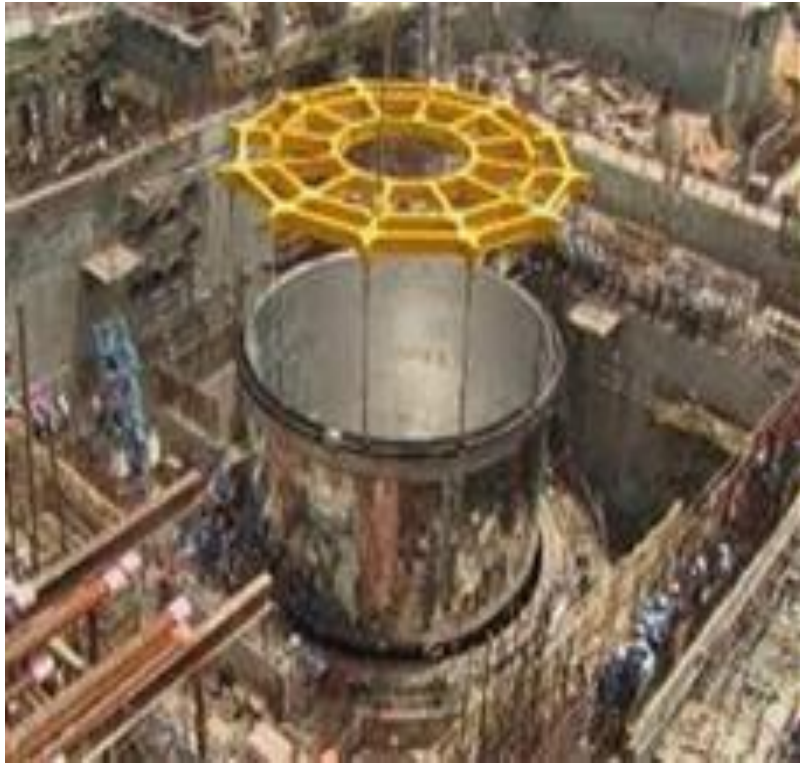
India's prototype fast breeder reactor under construction at Kalpakkam
