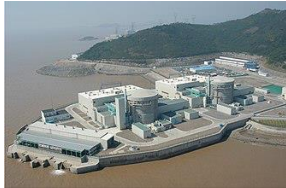
Two Candu-6 reactors (600 MWe each) at Qinshan
