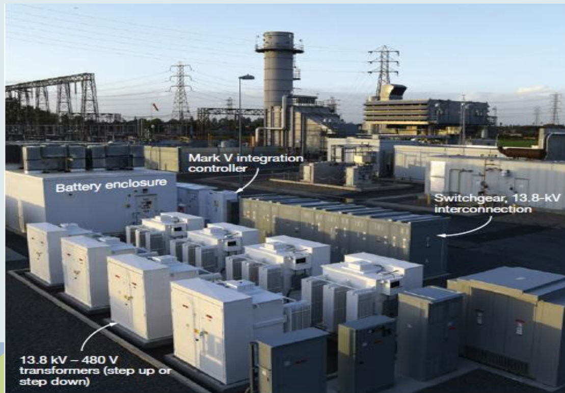
2. Center Peaker facility's battery dispatches power immediately upon receiving the CAISO dispatch signal and continues to provide power while the gas turbine/generator starts up
