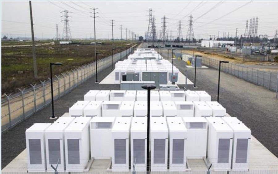
Flow battery, California, 2 megawatt 8 megawatt hours
