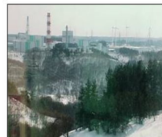
Rokkasho Uranium Enrichment Plant
