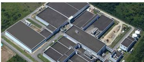
Rokkasho Uranium Enrichment Plant
