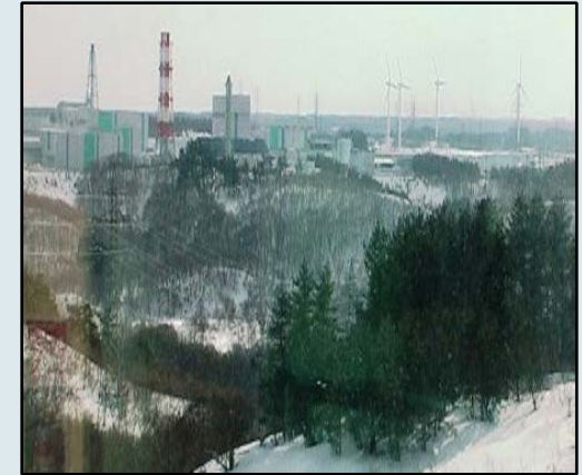
Rokkasho Uranium Enrichment Plant
