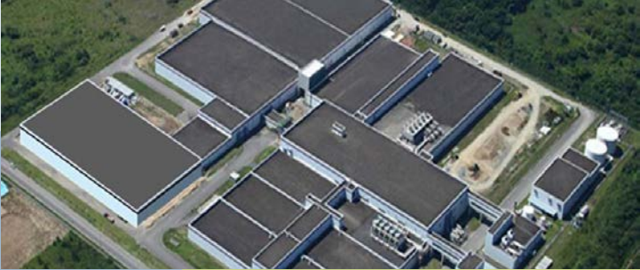
Rokkasho Uranium Enrichment Plant
